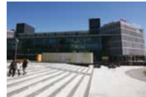
Spain PTA Malaga
